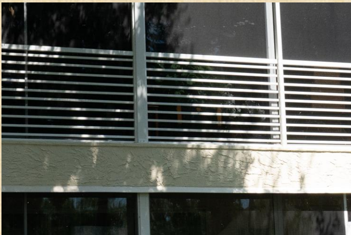
Rebuild with no flashing
