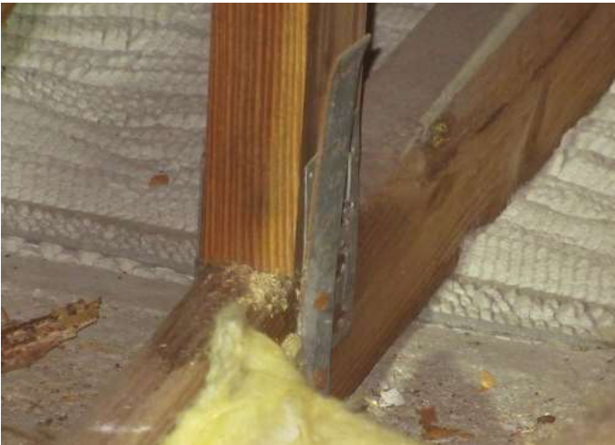
Single strap with 2 nails into the truss
