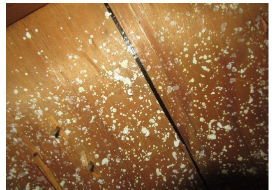
SWR installed under the roof covering
