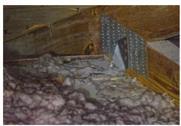
Clip with at least 3 nails into the truss
