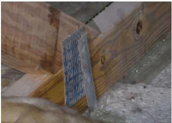
Single strap with 2 nails into the truss
