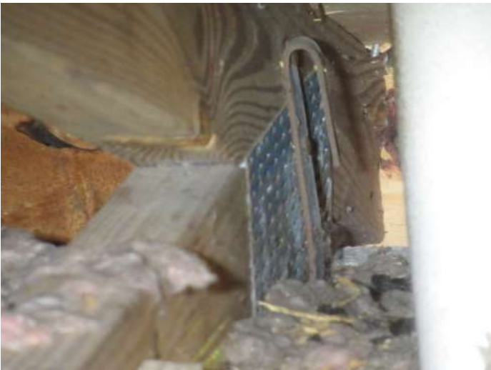
Single strap with 2 nails into the truss
