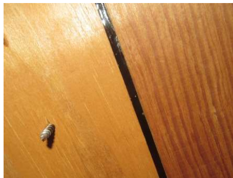
SWR installed under covering
