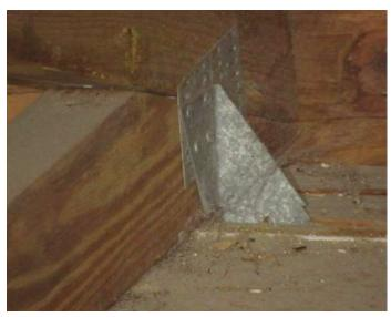
Clip with at least 3 nails into the truss
