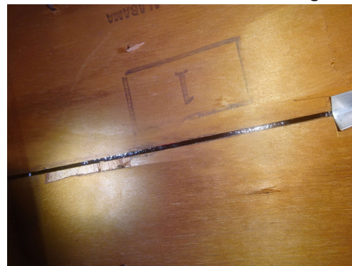
SWR installed under covering
