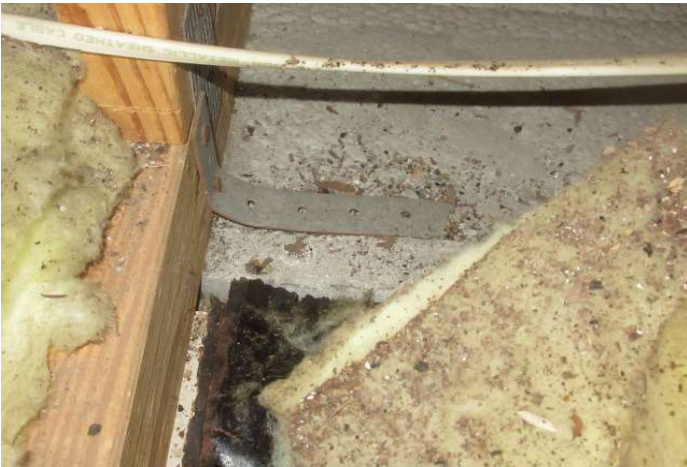
Single strap with 2 nails into the truss
