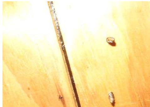
SWR installed under covering
