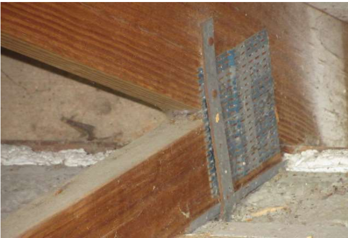
Single strap with 2 nails into the truss
