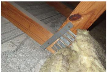
Single strap with 2 nails into the truss
