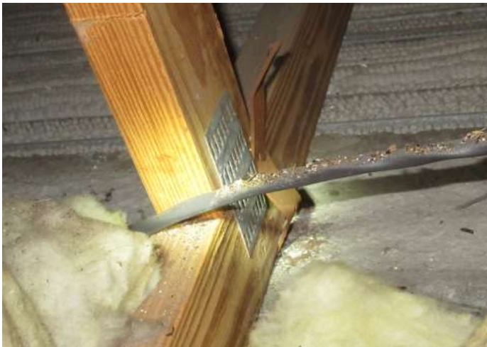
Single strap with 1 nail into the truss
