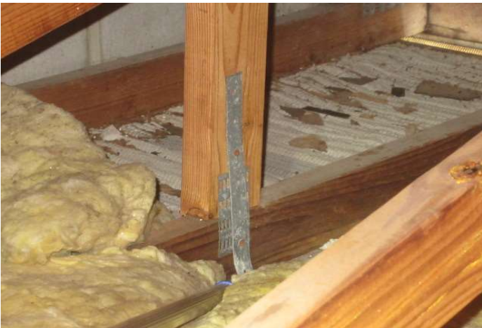
Single strap with 2 nails into the truss
